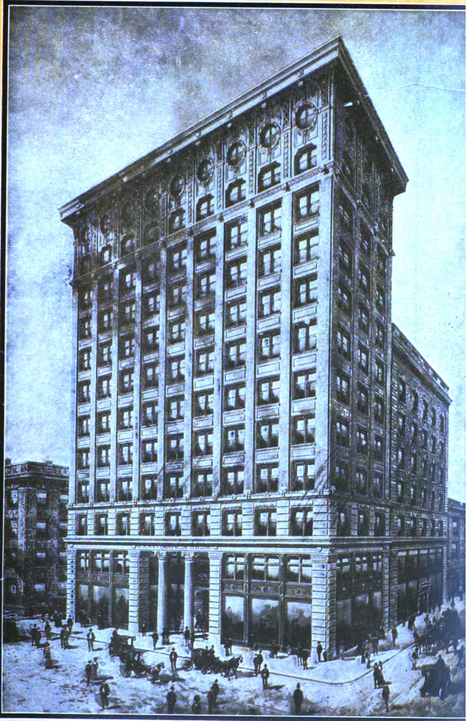
THE ALASKA COMMERCIAL COMPANY'S BUILDING, NORTHEAST CORNER OF CALIFORNIA AND SANSONE STREETS: WHITE GRANITE BASE AND GRAY TERRA COTTA SUPERSTRUCTURE; COST, ABOUT $500,000; ARCHITECTS, MEYERS AND WAI
